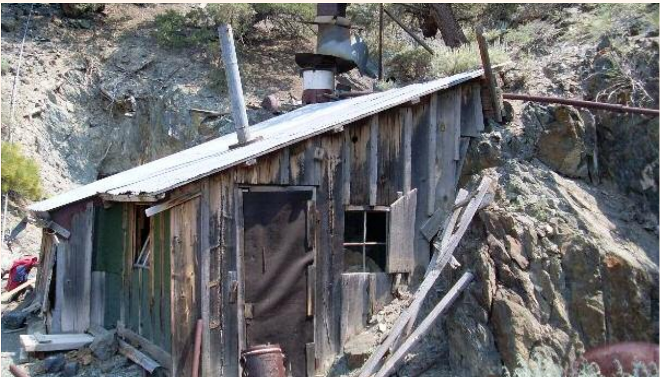
Miners cabin with wind generator (old washing machine and 50gal drum) to vent the adits and shafts.
